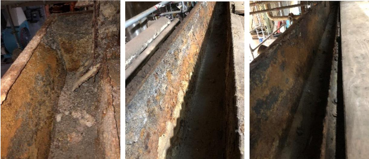
Helfrich will supply and install a new, 304 stainless steel water seal trough, 316 stainless steel saw tooth wear plate, 309 stainless steel baffle, scallop tube, air seals with gaskets and hardware, and W8 and C11 stiffeners. The replacement will involve removing and replacing a 2-foot band of 9-inch thick refractory around the entire perimeter of the bottom ash hopper.
