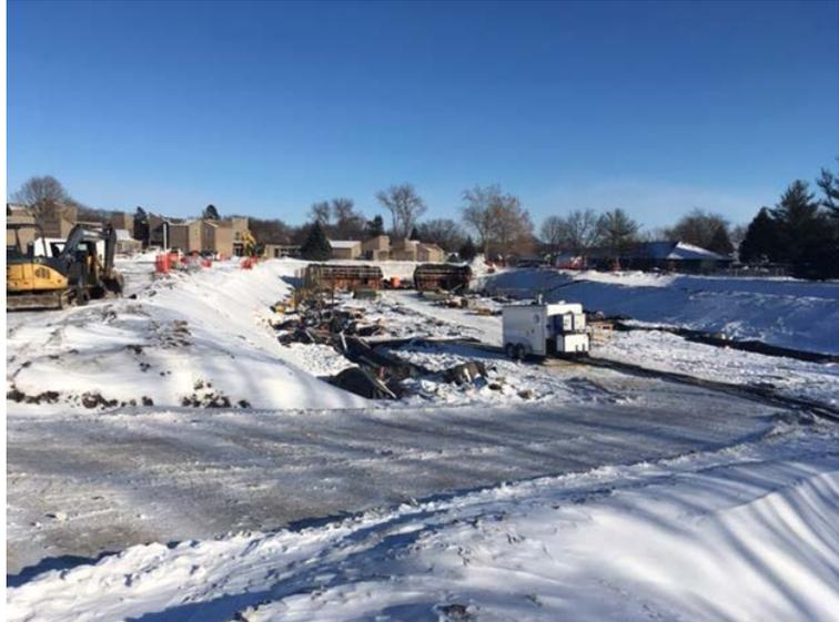
freezing before it can go through its full curing cycle. The Fire Department's Inspections Division has been busy helping the contractors stay on target with the project despite the cold temperatures. Inspectors ensure that footings meet engineering specifications and code requirements.
