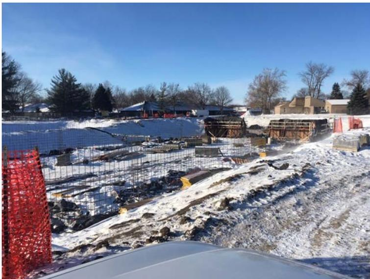
The next photo (left) was taken after the footings were approved and poured. The rebar has been placed into the footings, which will be inspected before the foundation walls are poured.
