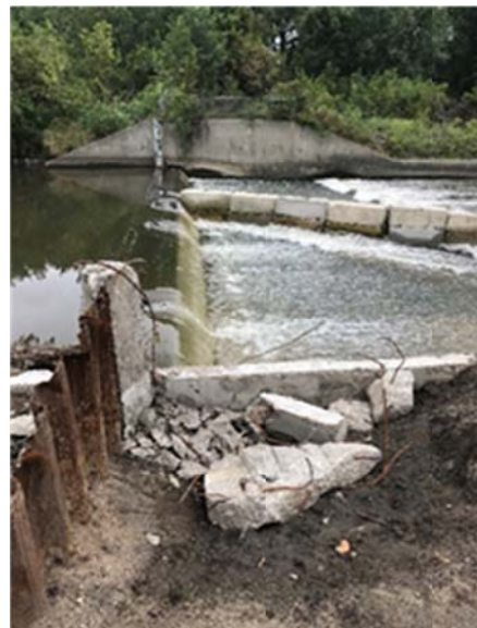
Construction work in progress on the low head dam.
