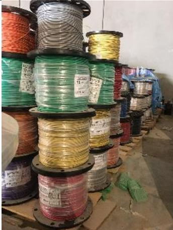
*Wiring for power and controls is underway. Each spool contains approximately one-half mile of wire.*
