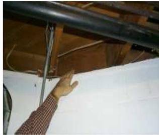
Cut fiberglass roll insulation into small pieces and place them into the rim joist spaces between the floor supports at the top of the outer basement walls.
