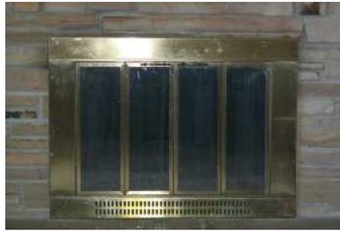
If you don't use a fireplace, consider adding board insulation to reduce heat loss or gain. Make sure the insulation is removed before any fire is built.
