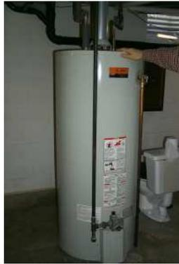
Newer water heaters have adequate insulation built into them. Older water heaters may benefit from the installation of a water heater insulation jacket. You may also save by installing insulation on the first 6 feet of hot water pipe. These products may be purchased at a hardware or lumber store.
