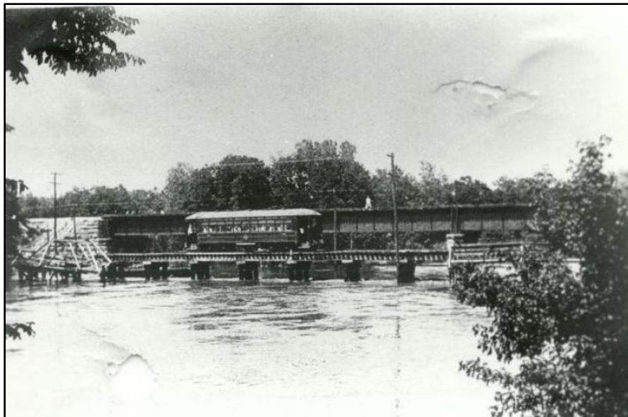
Figure 13. Remnant pieces of the foot bridge next to the streetcar on the left side, after it was washed away in the flood waters, 1918.
