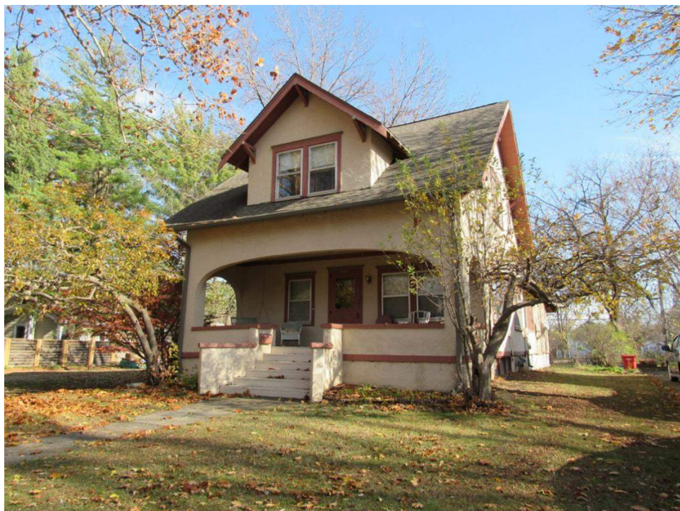
Photo 6. Façade of 926 Ridgewood Avenue, view to the northeast.
