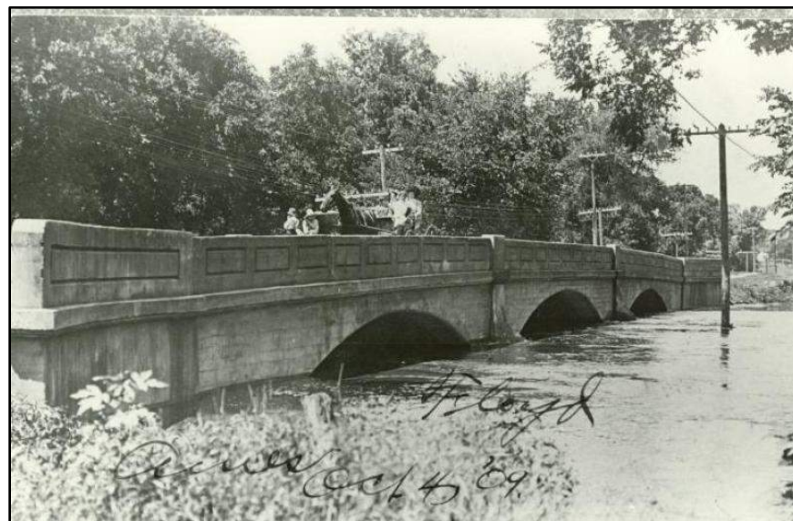
Figure 15. Lincoln Highway bridge over Ioway Creek. Within the year of construction, this flood water threatened the stability of the bridge, 1909.
