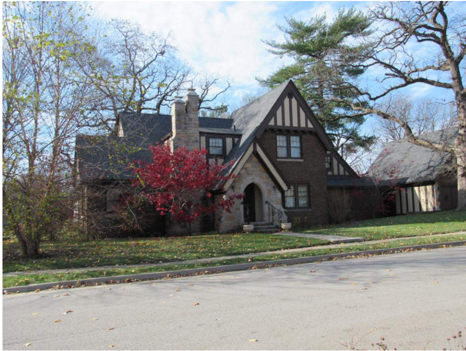
Photo 7. Façade of 1205 Ridgewood Avenue, view to the southeast.
