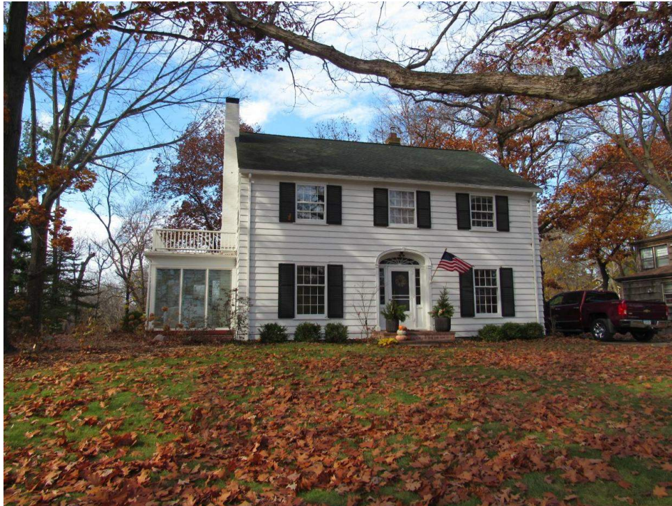
Photo 5. Façade of 1001 Brookridge Avenue, view to the northwest.
