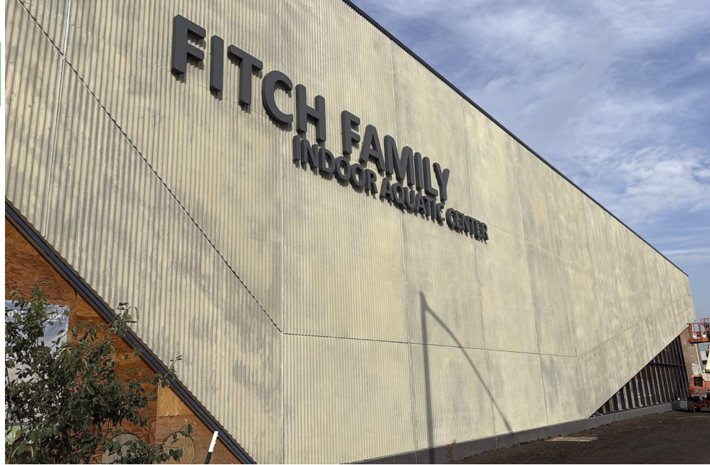
Precast South Elevation after Power Wash
