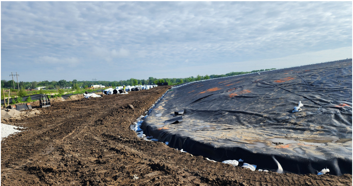
Photo 6 The southwest corner of the consolidated and capped area of the inactive impoundment showing geomembrane and anchor trench. Looking north. May 29, 2025.
