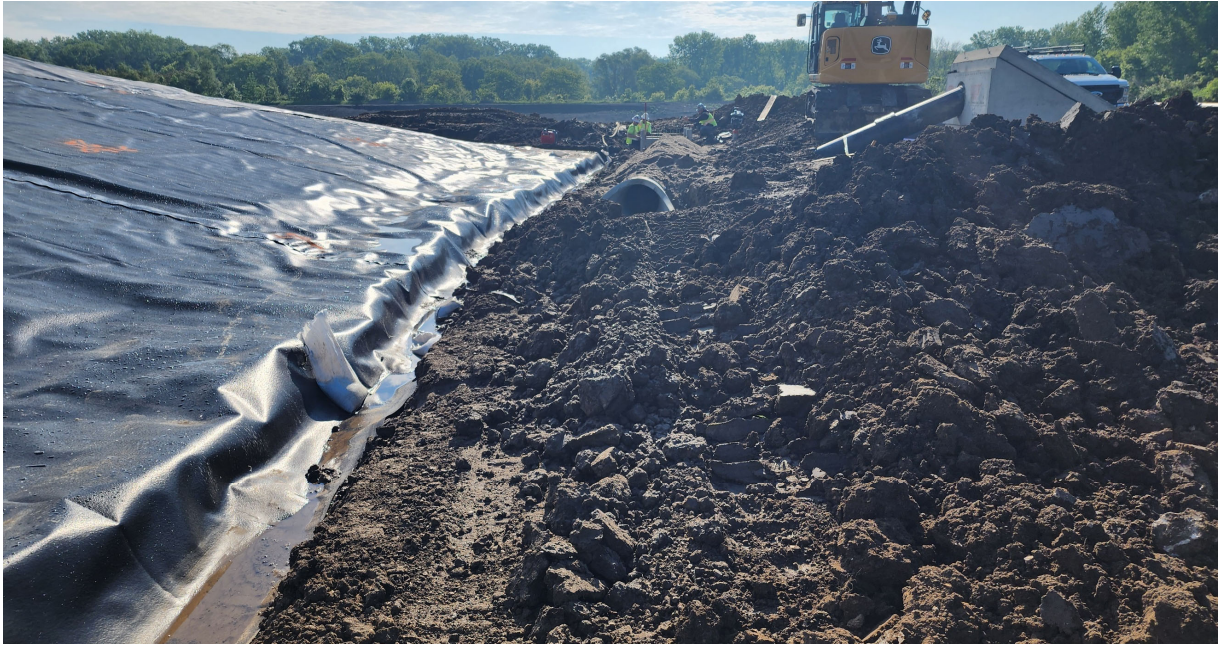
Photo 5 Portion of the southern perimeter of the consolidated and capped area of the inactive impoundment showing geomembrane liner and anchor trench. Looking east. May 29, 2025.
