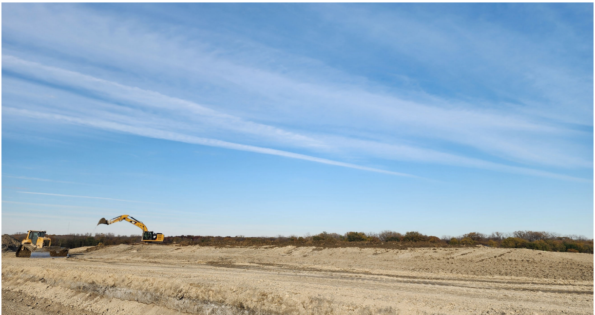
Photo 2 CCR grading and consolidation activities on the western portion of the inactive surface impoundment. Looking northeast. October 21, 2024.
