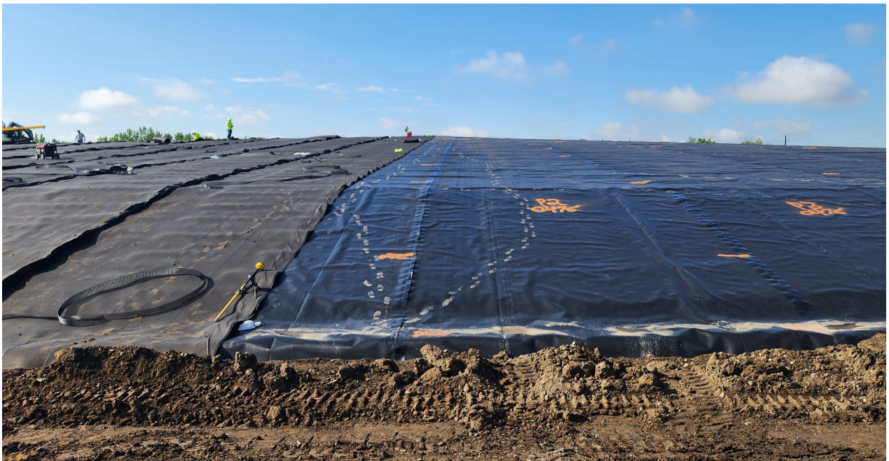
Photo 8 Installation of geocomposite drainage layer proceeding over geomembrane in the consolidated and capped portion of the inactive impoundment. May 29, 2025.
