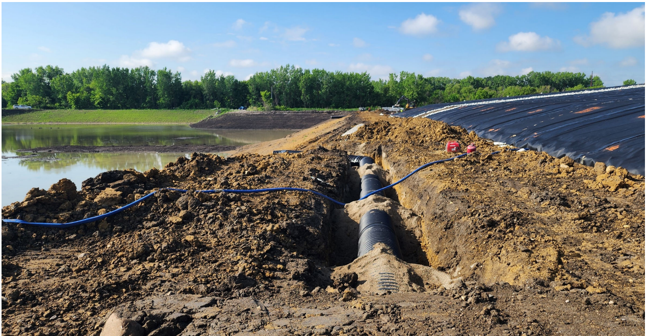
Photo 10 Stormwater management infrastructure in dividing berm between closed by removal area (left or east) and consolidated and capped area (right or west) of inactive impoundment. Looking south. May 29, 2025.
