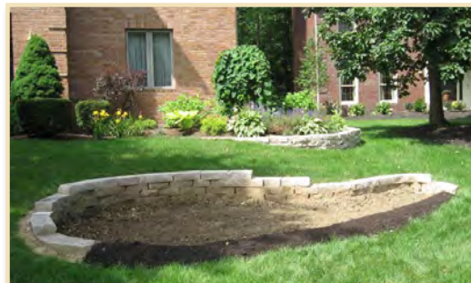
Upslope retaining wall around an oblong rain garden with a mulch berm on the downslope side.
