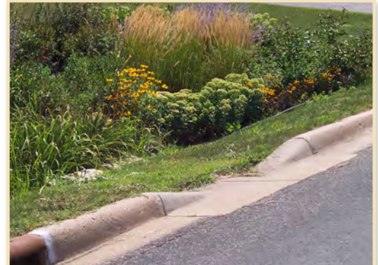
Grass filter strip used for pre-treatment area.
