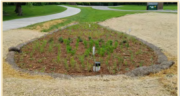
Enhanced rain garden with a vertical overflow structure.
