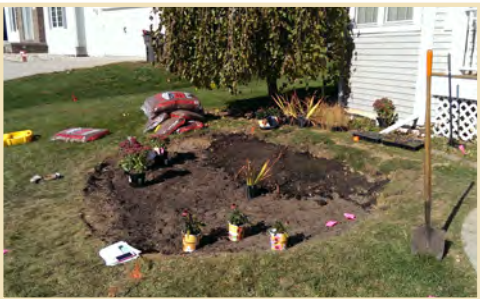
This rain garden was built below the yard surface with no berms. The water overflows onto the existing grass and flows away from the house.
