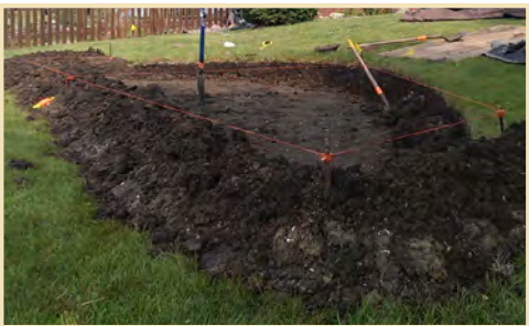
In order to achieve a ponding depth in the rain garden, this sloped site requires berms and/or retaining walls.
