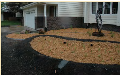
Rain garden berms under construction.
