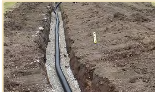
HDPE subdrain pipe in an enhanced rain garden.
