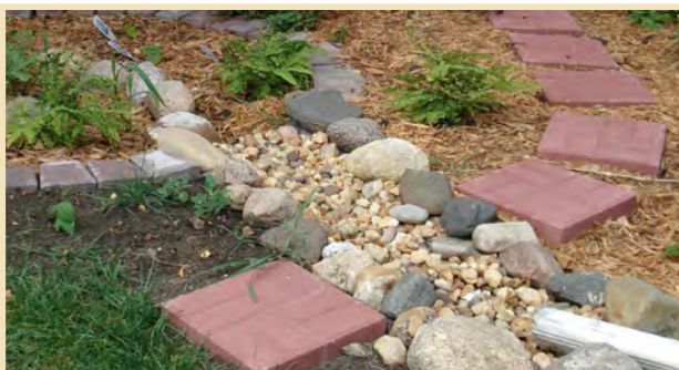
Gutter extension added to downspout to move rainwater to rain garden.
