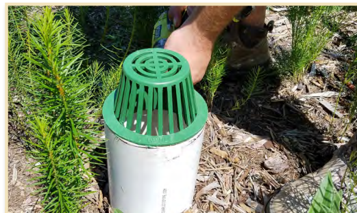
Overflow structure extending to the top of the ponding depth.
