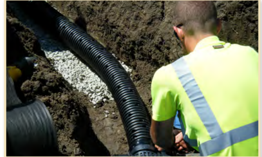
Placement of perforated subdrain.
