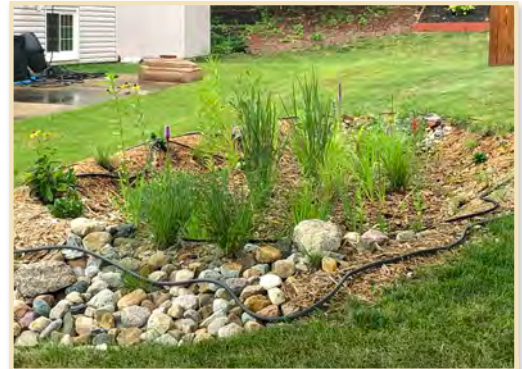
Using a soaker hose for watering in a new rain garden.
