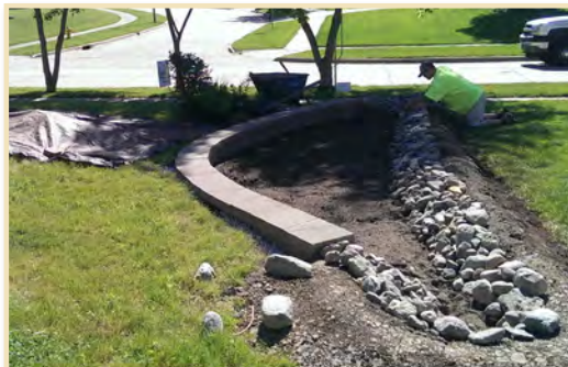
Rain garden under construction.
