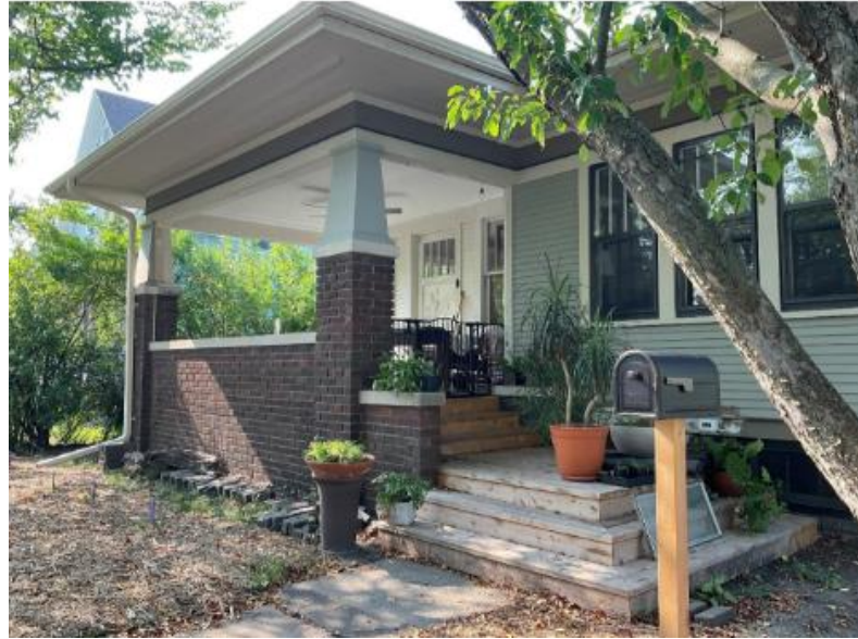
723 9 th – Porch Restoration
