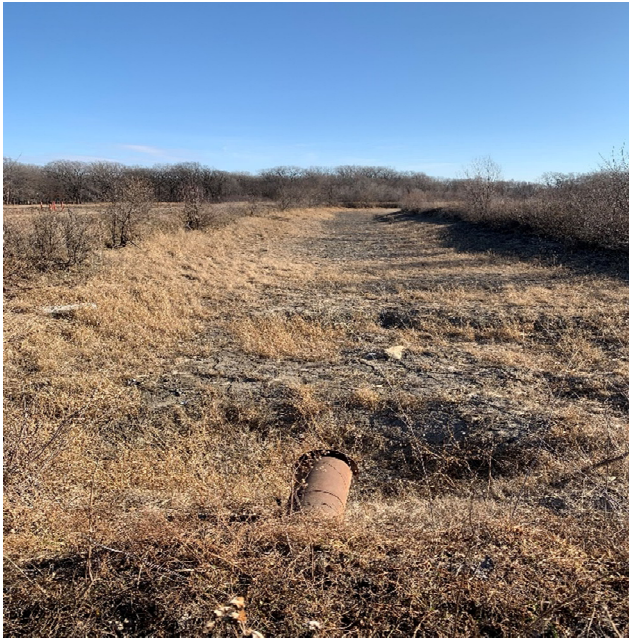
Photo 29: 2021 SEP floor drain and cooling tower blowdown discharge pipe into the north side of north storage area in the ash pond.
