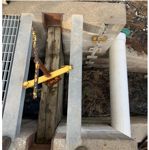
Photo 14: 2022 Gauge located at ash pond outlet structure (AP-1)
