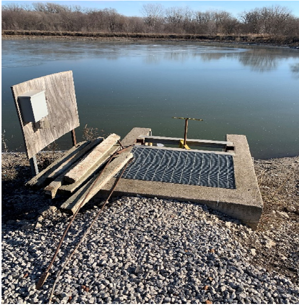
Photo 9: 2021 Ash pond outlet structure
