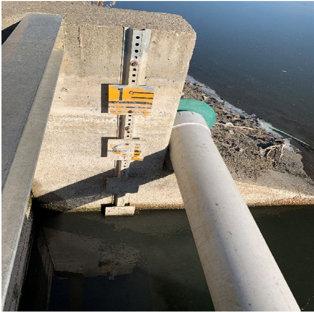
Photo 13: 2021 Gauge located at ash pond outlet structure (AP-1)
