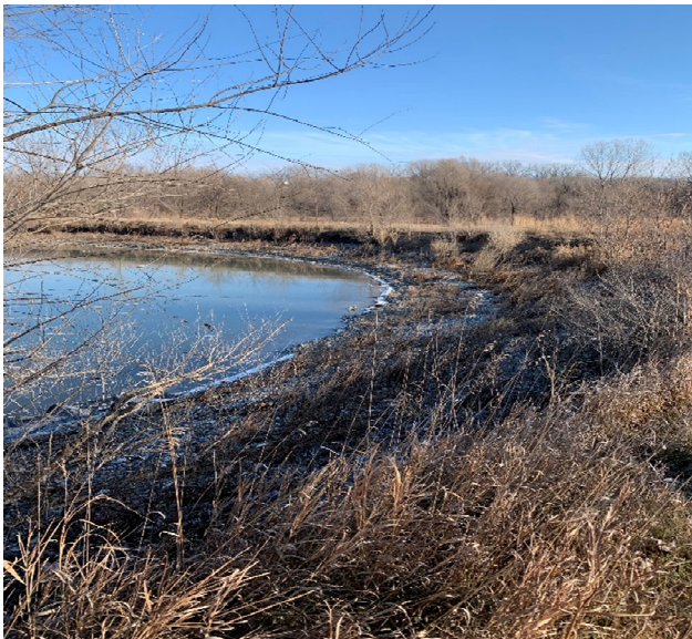
Photo 7: 2021 Erosion along inside slope south embankment
