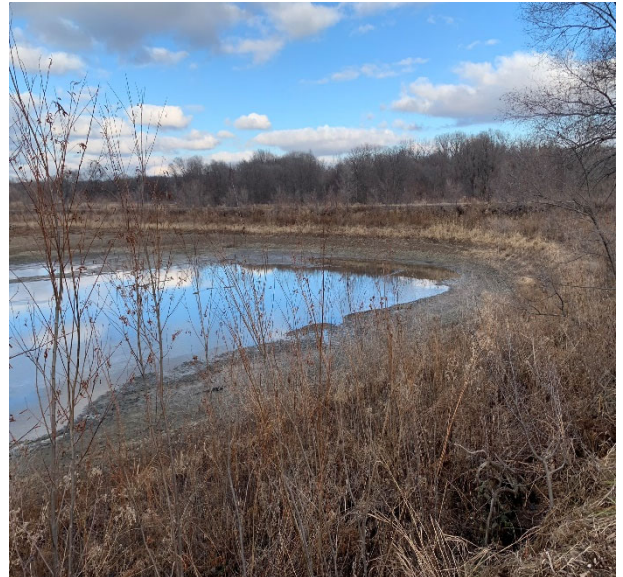
Photo 8: 2022 Erosion along inside slope south embankment
