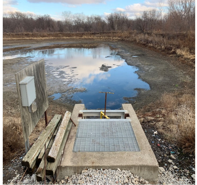
Photo 10: 2022 Ash pond outlet structure
