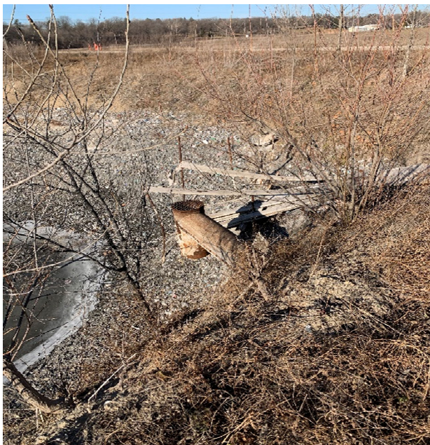
Photo 27: 2021 Pipe structure connecting west channel to northern area in the ash pond.
