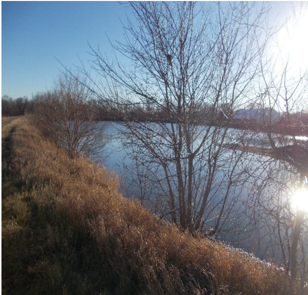
Photo 17: 2020 Example of vegetative growth to be removed on northeast corner of the ash pond.
