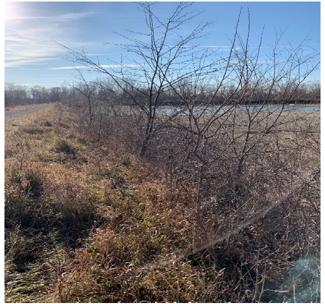
Photo 18: 2021 Example of vegetative growth to be removed on northeast corner of the ash pond.
