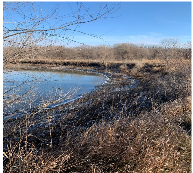
Photo 8: 2021 Erosion along inside slope south embankment
