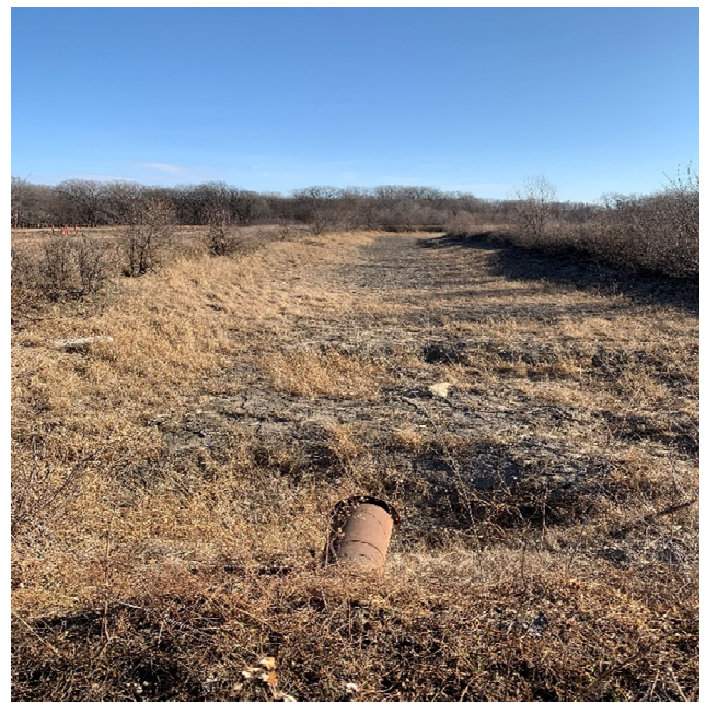
Photo 30: 2021 SEP floor drain and cooling tower blowdown discharge pipe into the north side of north storage area in the ash pond.
