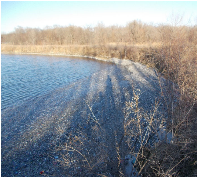
Photo 7: 2020 Erosion along inside slope south embankment
