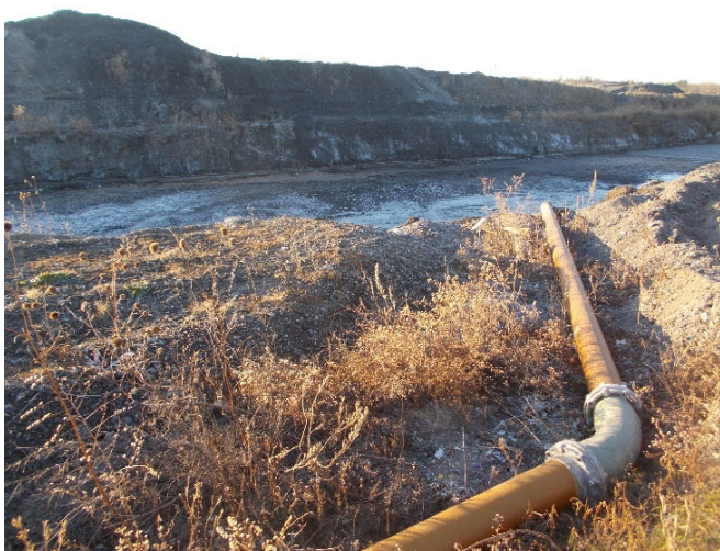
Photo 23: 2020 Ash sluice pipe to West Ash Pond Receiving Ditch
