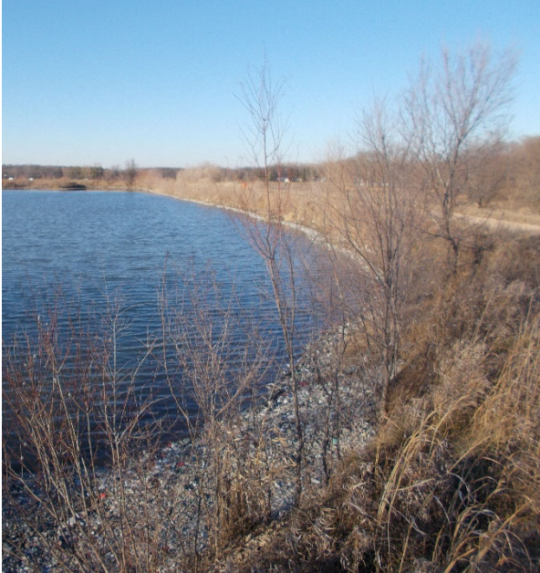
Photo 21: 2020 Erosion on inboard slope southeast portion of the ash pond from south looking northeast. See Area 2 for location.
