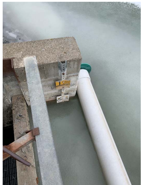
Photo 16: 2019 Gauge located at ash pond outlet structure (AP-1)
