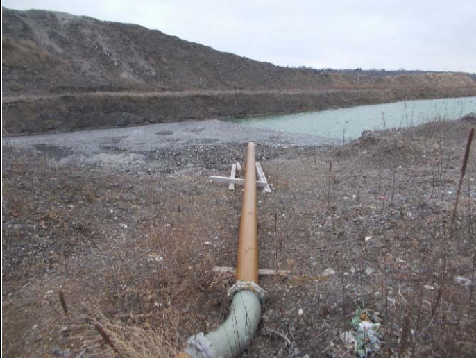
Photo 25: 2018 Ash sluice pipe to West Ash Pond Receiving Ditch
