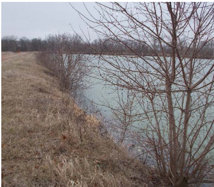
Photo 19: 2018 Example of vegetative growth to be removed on northeast corner of the ash pond.
