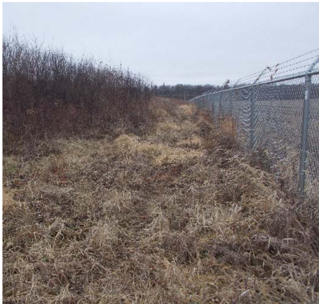
Photo 9: 2018 Outside slope north embankment viewing west. New fence and vegetation needing removal.
