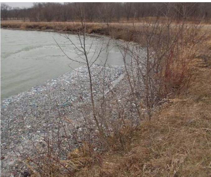
Photo 7: 2018 Erosion along inside slope south embankment
