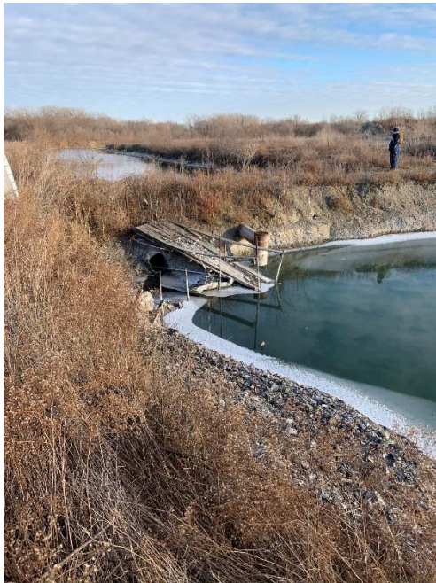
Photo 29: 2019 Pipe structure connecting west channel to northern area in the ash pond.
