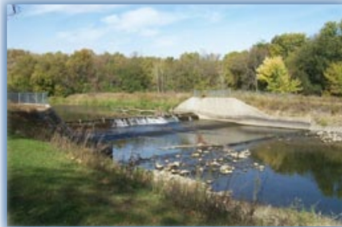
The low-head dam aids in recharging the downtown aquifer.
