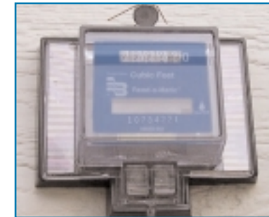
This device on the outside of your house communicates the reading from your water meter to the meter reader
