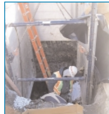
Repairing water main beneath the street
